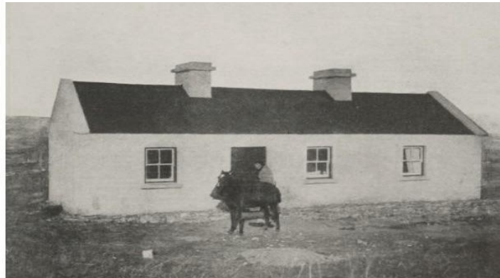
The new houses (images reddit.com)
