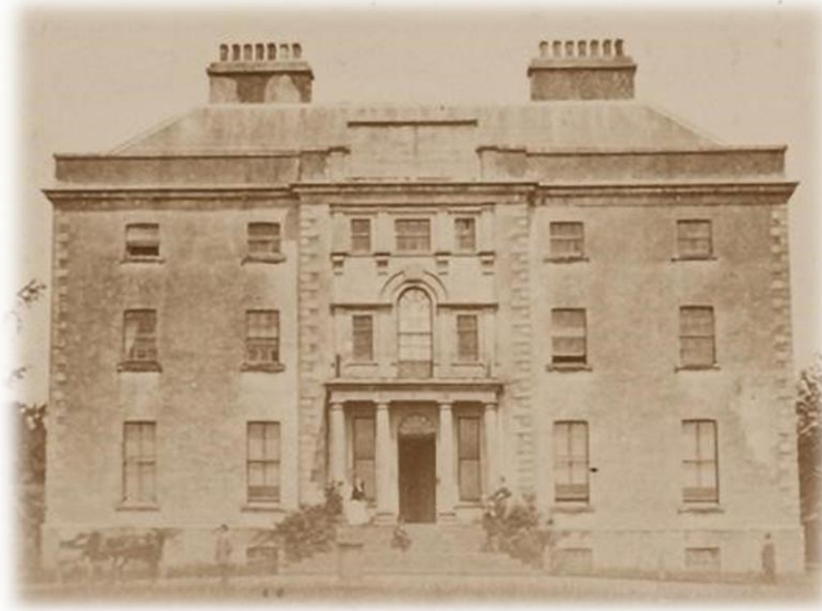
Moore Hall as it originally looked ( buildingsofireland.ie )
